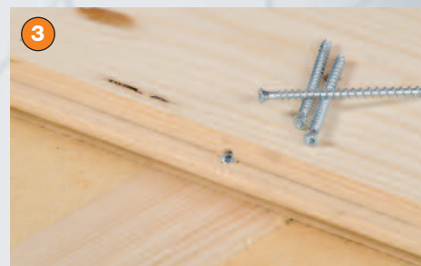
3 Gap free axial fixing of the timber board via the HECO-UNIX full thread
