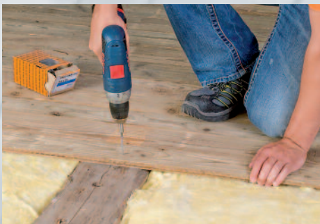
Floor board fastening
